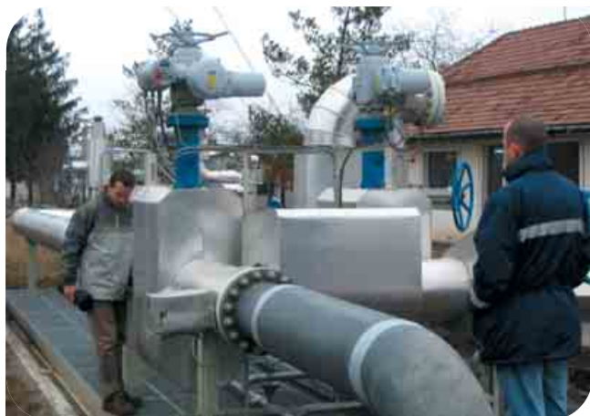
Intelligent actuators on metering skids Oil pipeline (Romania)
